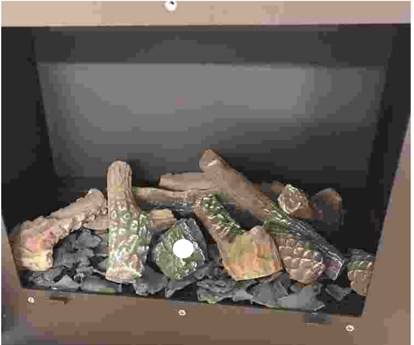
Step 10 - Position Ceramic Log 5 so it sits at the front – as per the picture above – As marked with the White Dot
