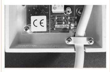
Carefully fit the control plate into the back box ensuring that no wires are trapped during the sitting process.
